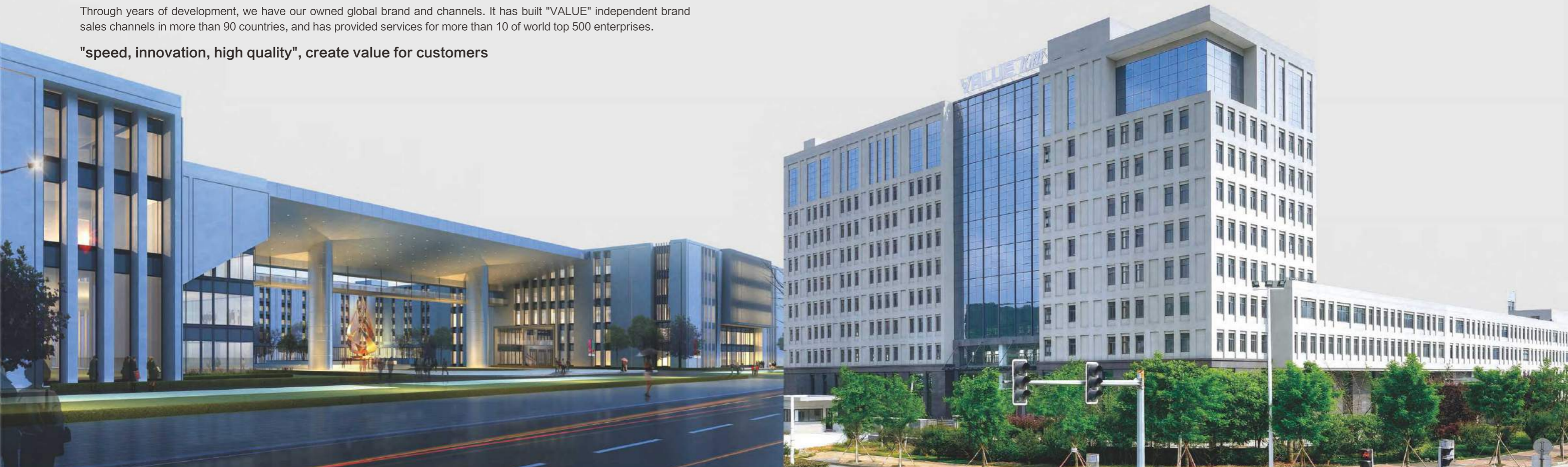
The third production base, a new smart factory is under construction
