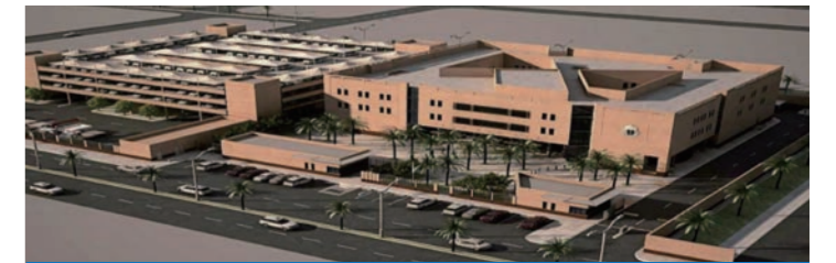
KAP 4 & 5 Project, KSA
