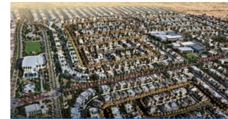
Ajyal Aramco Dhahyal Housing, KSA
